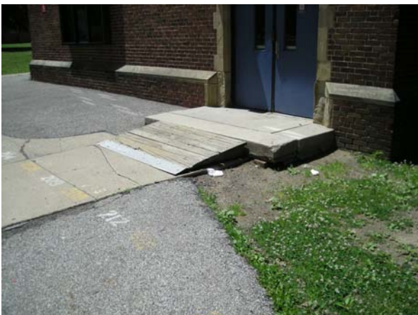
Noncompliant Wheelchair Entry Ramp
