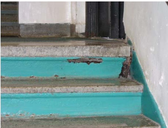
Corrosion on Metal Stairs
