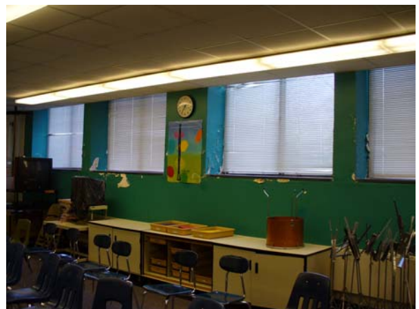
Water Damage in Music Room
