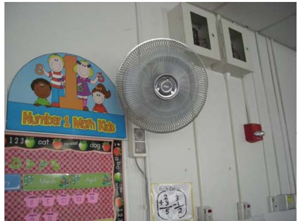
Wall Mounted Classroom Fan
