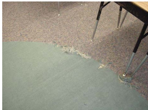
Frayed Classroom Carpet
