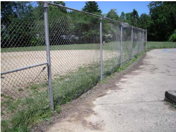
Typical Condition of Site Fencing
