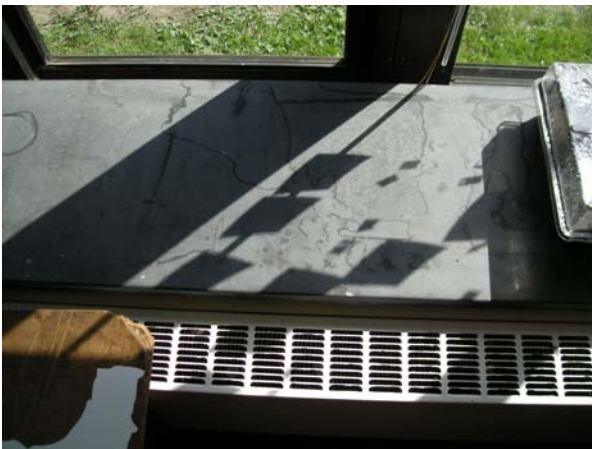
Fin Tube Enclosure at Windowsill
