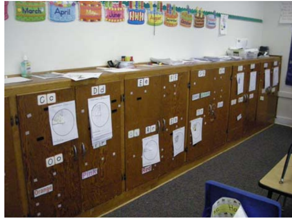
Obsolete Casework in Kindergarten
