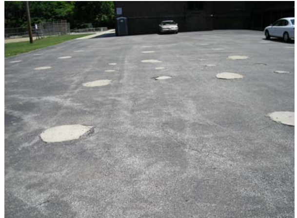
Patches in Bus Parking
