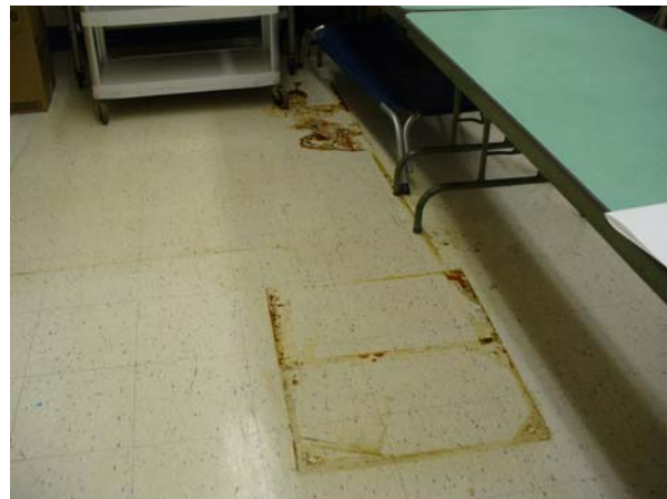
Damaged Kitchen VCT
